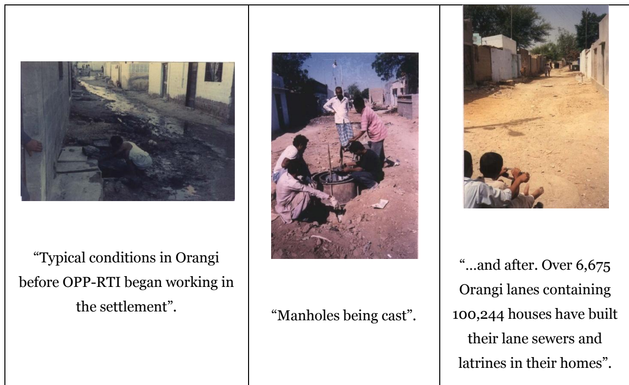
Figure 4: Photographs from Orangi Pilot Project (Orangi Pilot Project (OPP) - Institutions and Programs, 2009).
