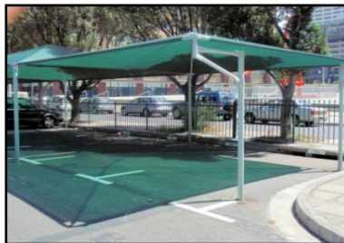
Figure 11: Permanent, galvanized steel framed canopy
