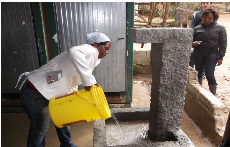
Figure 8: Co-Researcher Nyameka Using the Foot Operated Tap
