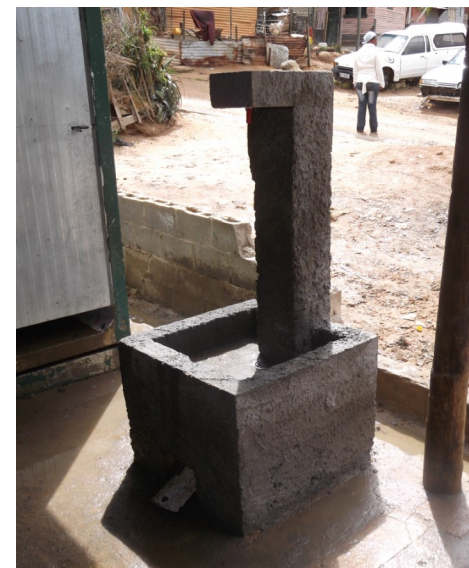
Figure 9: Foot Operated Tap
