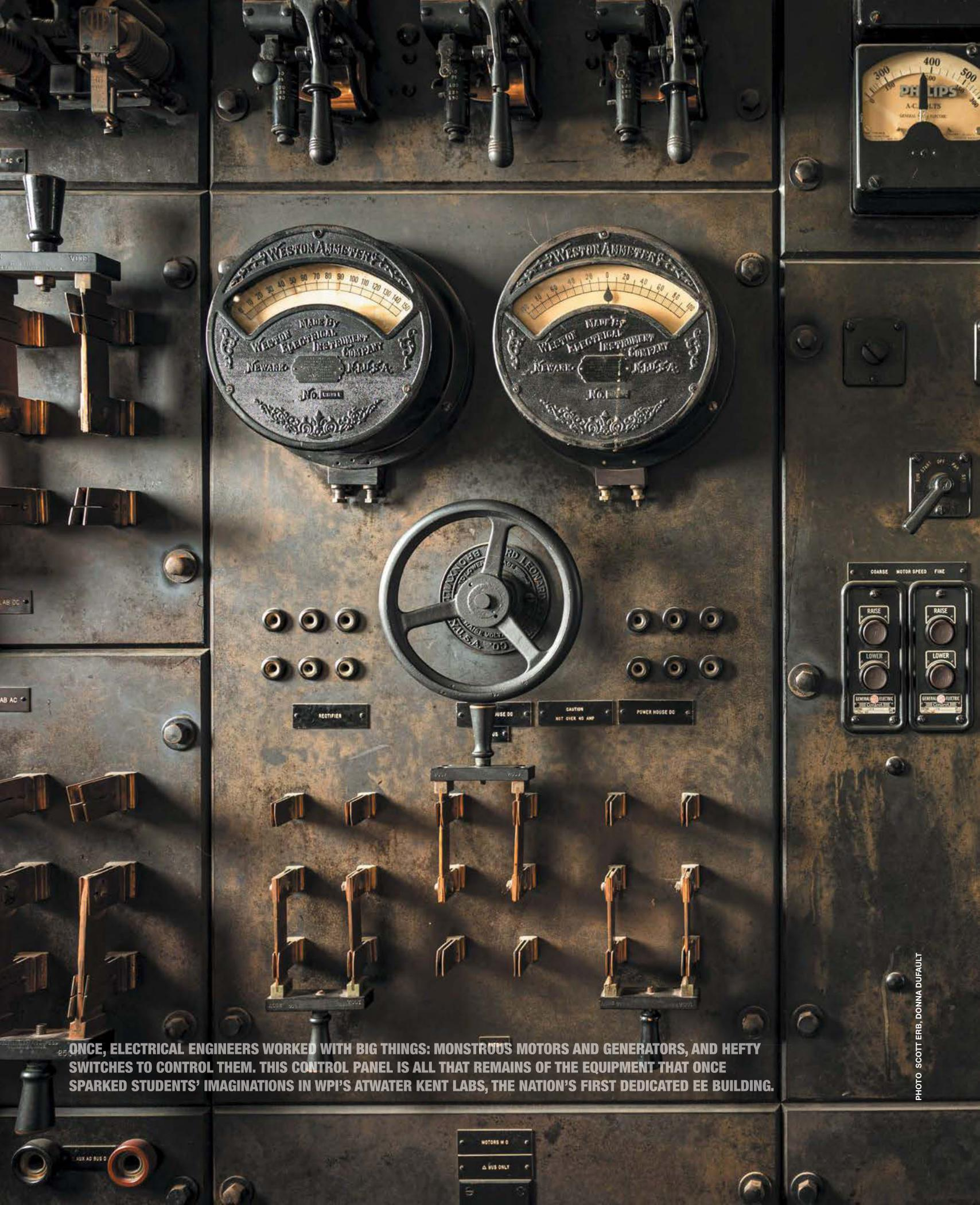
ONCE, ELECTRICAL ENGINEERS WORKED WITH BIG THINGS: MONSTROUS MOTORS AND GENERATORS, AND HEFTY SWITCHES TO CONTROL THEM. THIS CONTROL PANEL IS ALL THAT REMAINS OF THE EQUIPMENT THAT ONCE SPARKED STUDENTS' IMAGINATIONS IN WPI'S ATWATER KENT LABS, THE NATION'S FIRST DEDICATED EE BUILDING.
