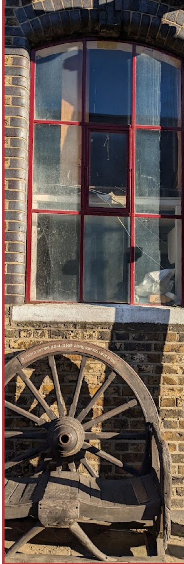
Outside of the Main Pumphouse
