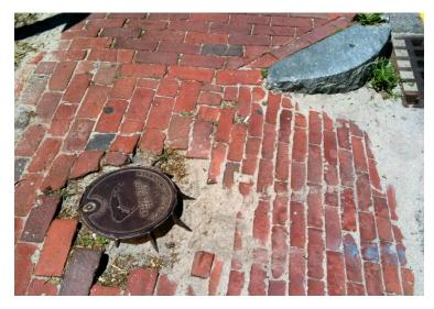
Figure 2.4 Example of Uneven Footing (Island Oracle, 2015)
