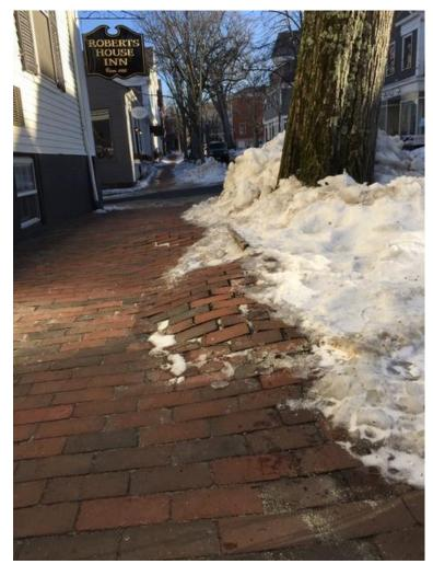
Figure 2.3 Example of Tree Roots Damaging the Brick Sidewalk (SeeClickFix, 2015)
