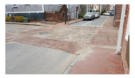
Figure 4.6 Example of a 4-way intersection that meets ADA standards (North Union St. and Cambridge St.)
