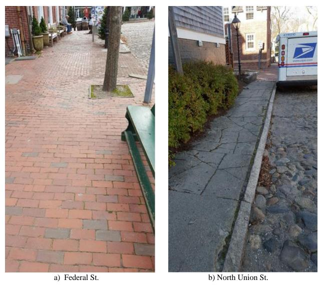
Figure 4.2 Example of a sidewalk given a) a rating of 1 versus a sidewalk given b) a rating of 4
