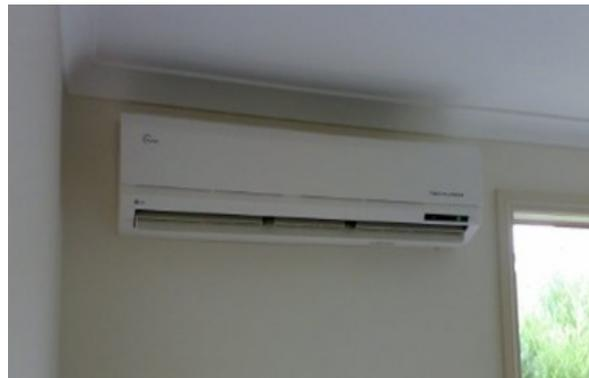
**Figure 5. Fully installed reverse cycle air conditioning unit**
