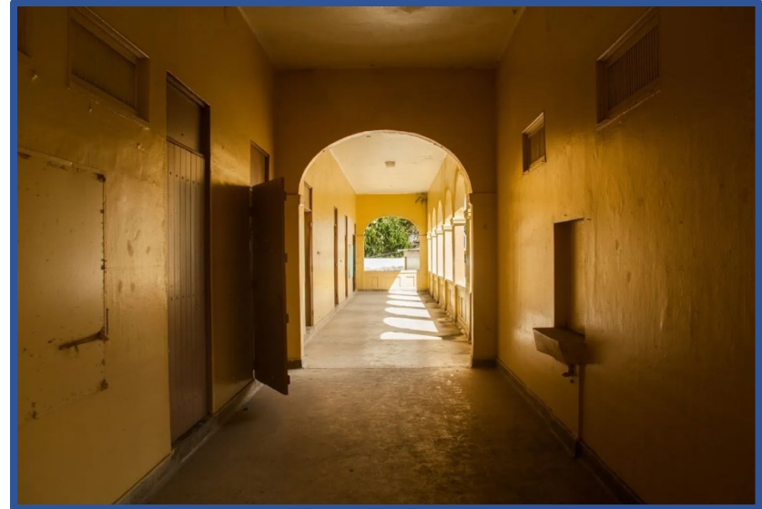
Figure 12: Photo of empty hallway in Pedro G. Elementary School (Donelly-DeRoven, 2019).
